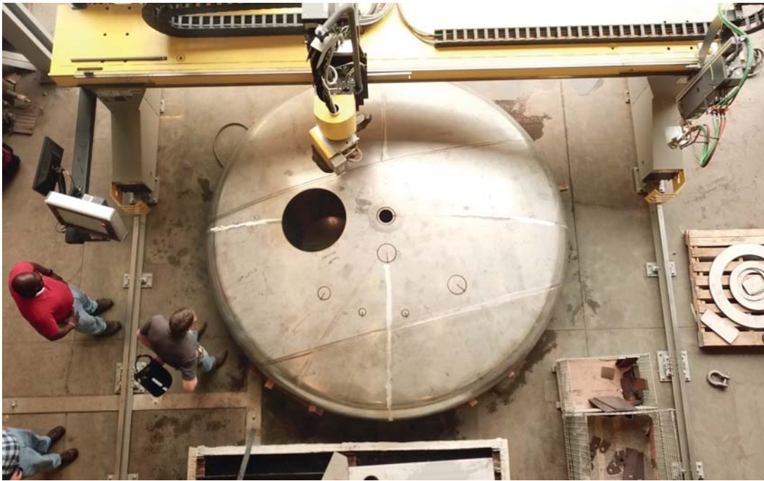
➤ Innovation- burning holes with prepped weld bevels in heads.
