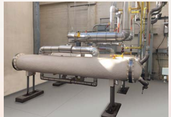
⚡ Patented thin-film SX ammonia-wine evaporator for a winery plant
