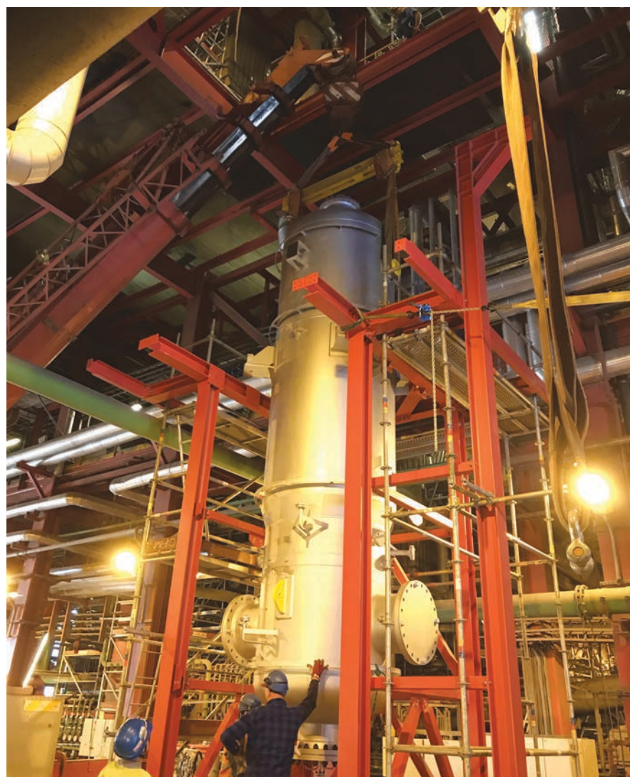
Customized heat exchanger from Hexonic working in the heating system and supplied with steam from the reduction and cooling station. Its role is to heat up the district water to the set parameters during the peak heat demand in winter periods.
