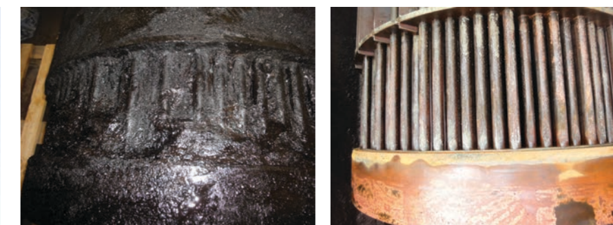
Before (left) and after (right) of a straight bundle heat exchanger through thermal cleaning.
