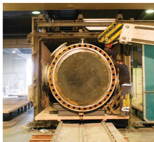
➤ Preparing a 32 ton heat exchanger for thermal cleaning.
